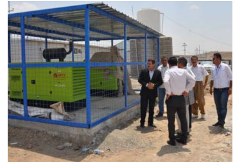
Installation of power generators at Kawirgosik Syrian refugee camp
